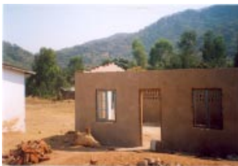
Library construction at Monkey Bay Primary School
