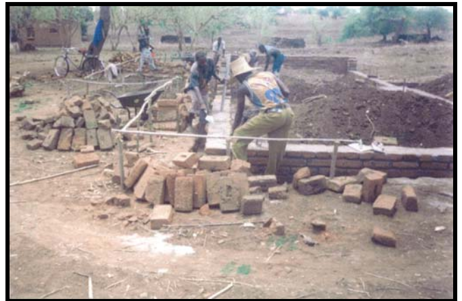
Construction in progress on Chizungu Community Library
